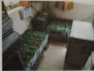
Batteries stacked for disposal
